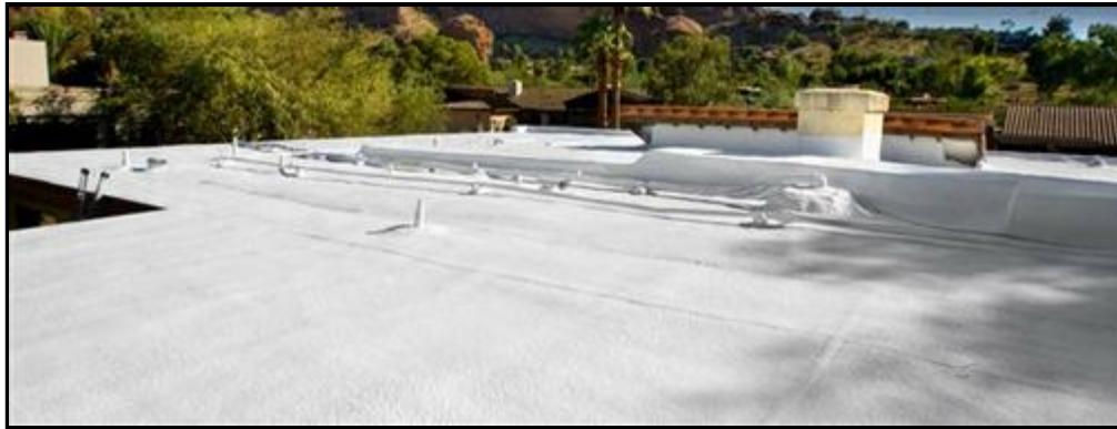
1.0 Picture 13 Bayblock roof coating
