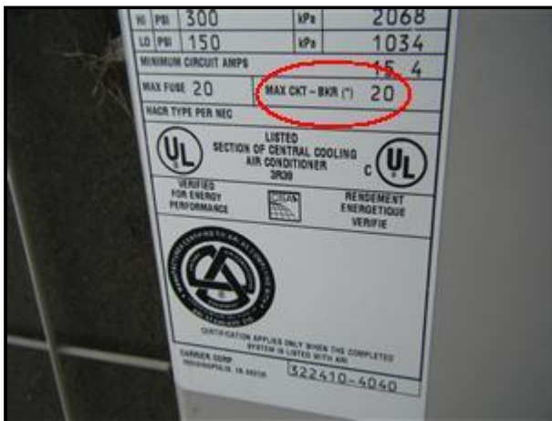
8.6 Picture 4 Max Breaker 20 Amp
