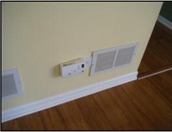
7.8 Picture 1 Plug-in CO detector
