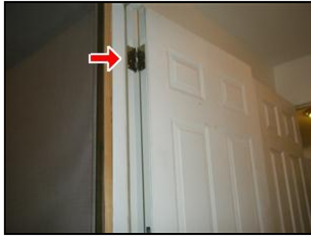
3.6 Picture 1 Install spring hinge or closer
