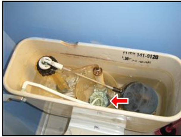
6.1 Picture 4 Master bath toilet
