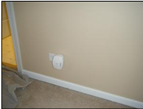
7.8 Picture 3 Plug in CO detector on 2nd floor
